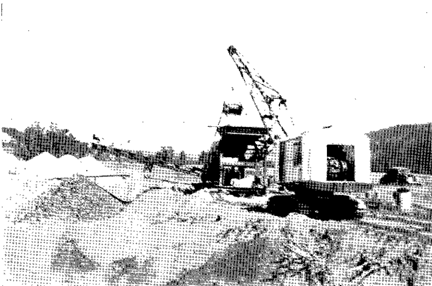
Mobile digging and sluicing plant of Canamco, Ltd., in operation on Fraser River, 5 miles above Quesnel.
