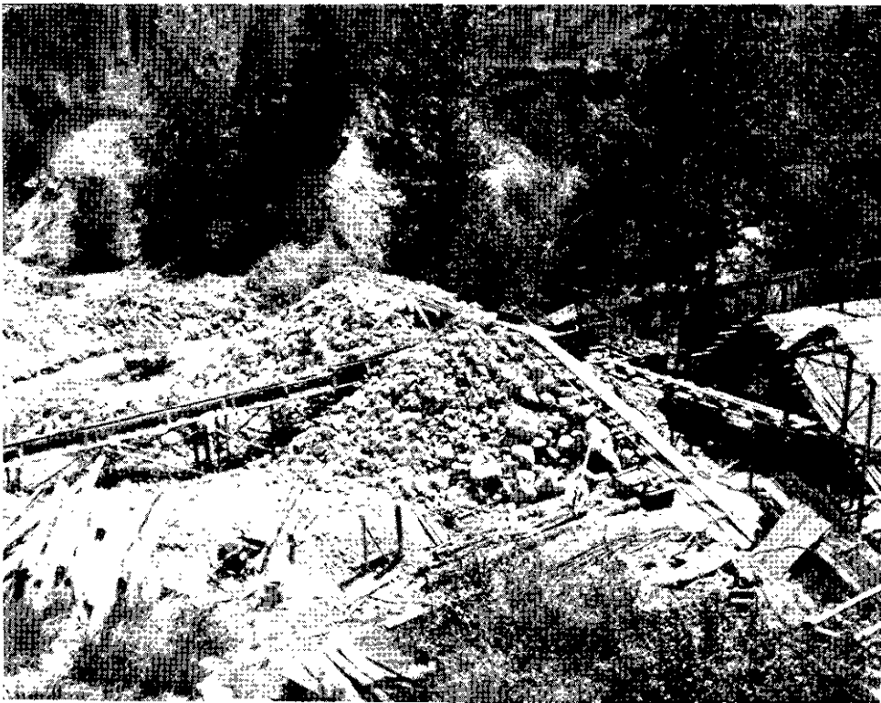
Upper Jolly Creek. Incline track from drift workings.
