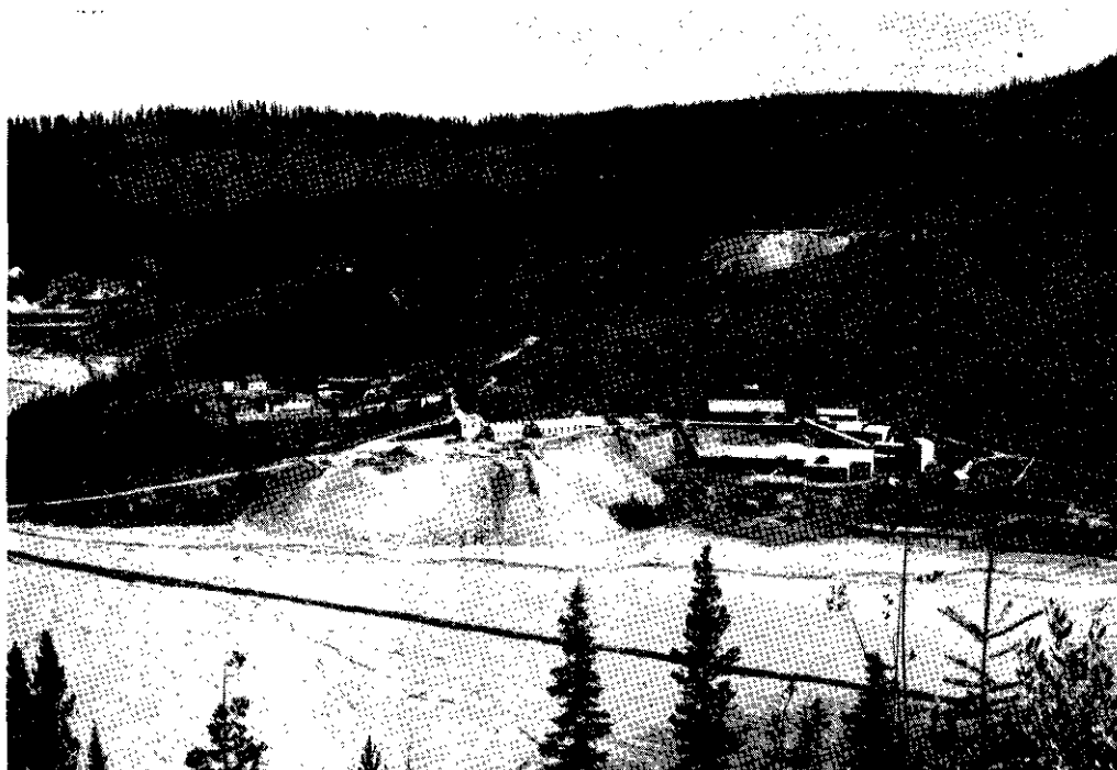
A. View of Cariboo Gold Quartz mine from Island Mountain, showing the camp to the left of the 1500-level dump and the power-house and mill to the right; the 1200-level dump is at the upper right; Lowhee Creek is in the left background; and tailings from the Lowhee hydraulic are in the foreground.
