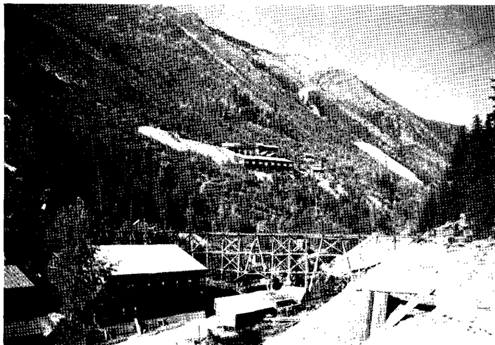
B. Sheep Creek Valley with Gold Belt mill in centre distance and Kootenay Belle mill in foreground.
