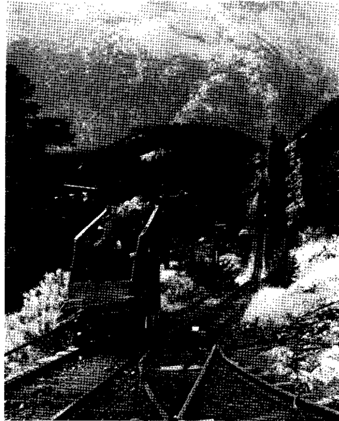
B. Six-ton ore skip on surface tramway, Nickel Plate mine, Hedley.
