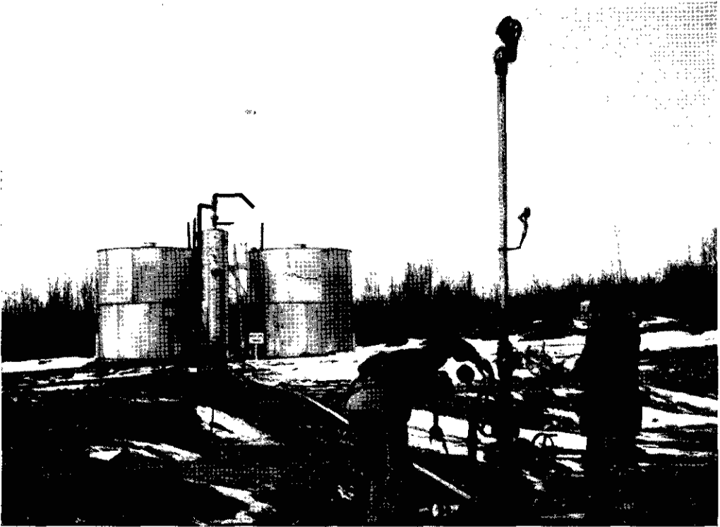
Running pressure test at well-head, Pacific Imperial Boundary Lake 1. Separator and storage tanks in background.
