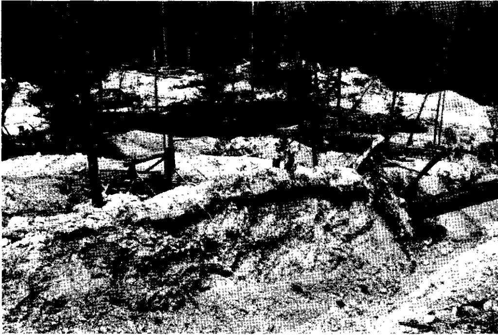
Bethlehem Copper Corporation Ltd., Highland Valley. Bulldozer stripping near an old shaft on a molybdenite-copper showing.
