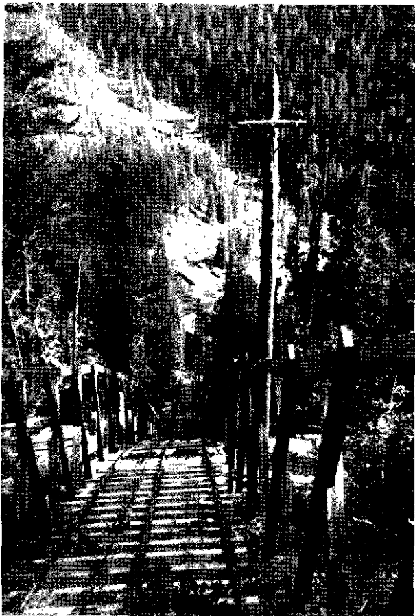
Mastodon skipway leading from mill on La Forme Creek to narrow-gauge railway.
