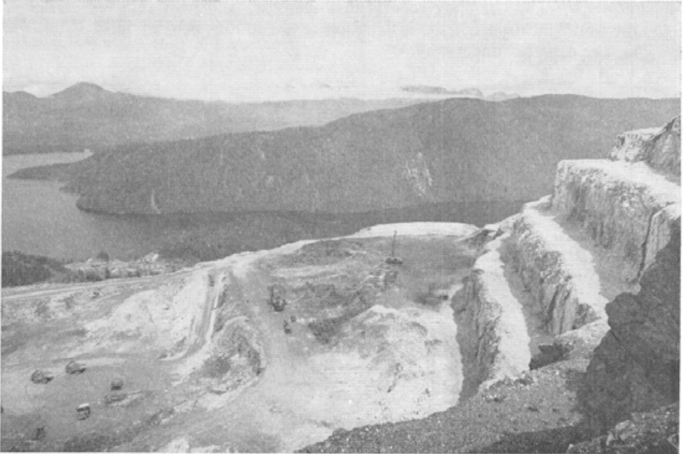
Plate VIA. Open pit at Tasu mine, Moresby Island.
