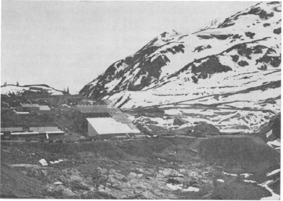
Plate IA. Granduc mine, looking south to mill under construction and portal of Granduc tunnel in June, 1968.
