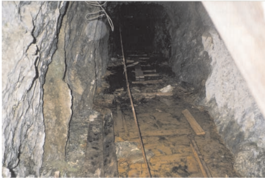
Photo 46. Camborne adit. The mine water was stagnant when sampled.
