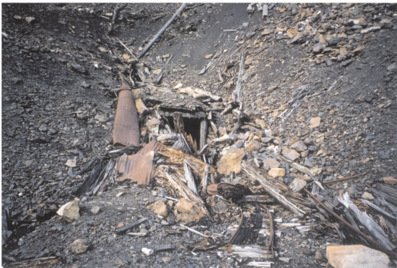
Photo 48. Jackson adit (elevation 1760 m). The drainage flowing from the adit is not visible in the photo.
