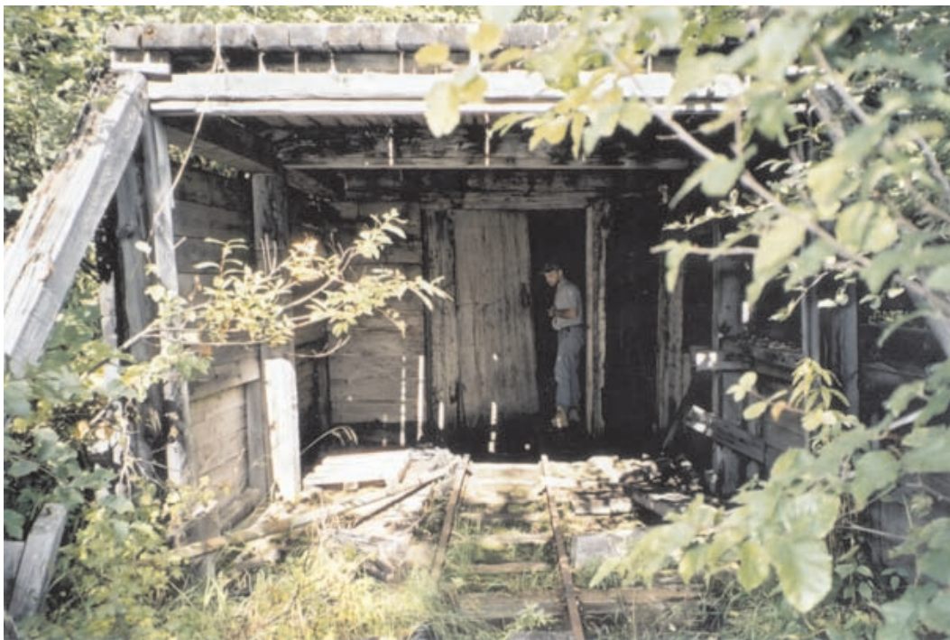
Photo 50. Slocan Sovereign adit with flowing drainage.
