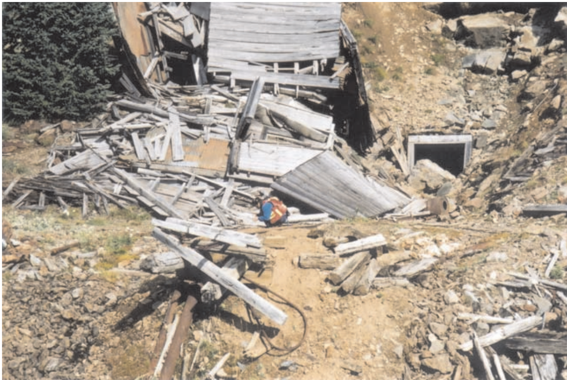
Photo 52. Lower adit. The drainage from the adit is being sampled.
