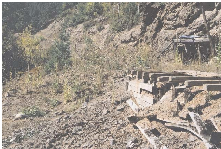
Photo 16. Congress adit (background). The drainage from the adit is draining from a small pipe, located below the tracks.
