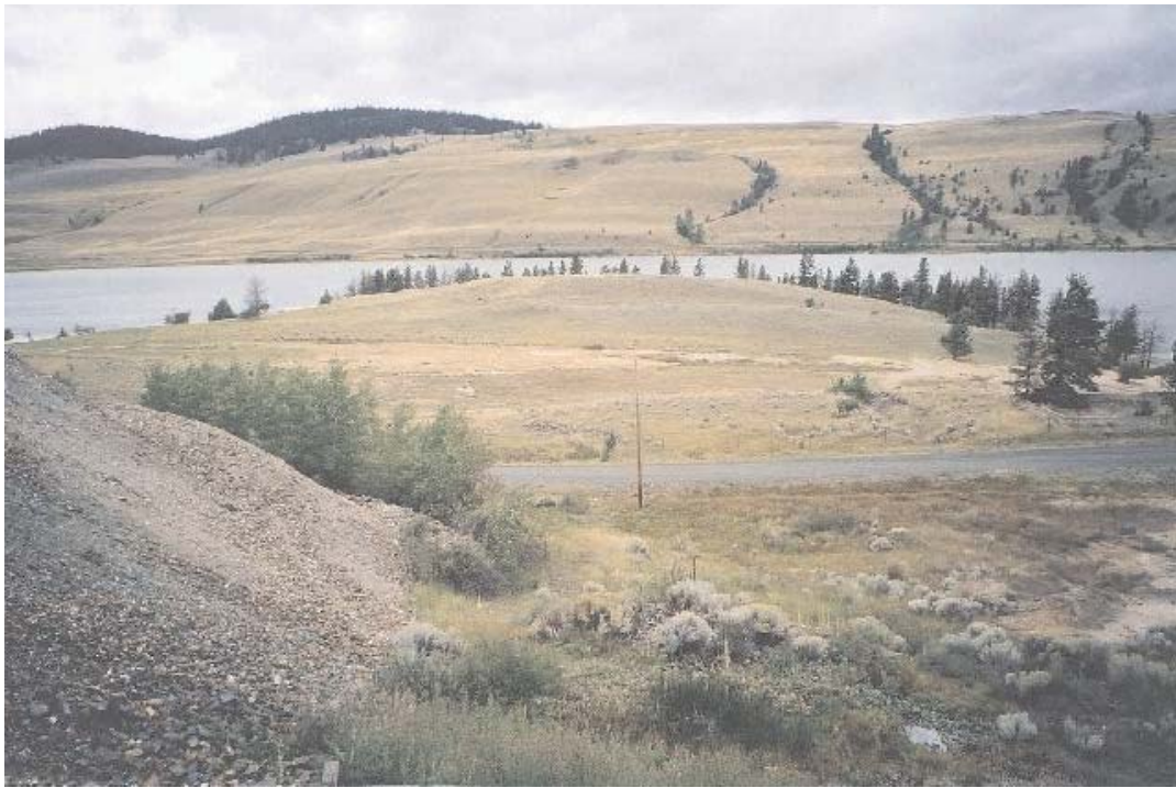
Photo 26. The partially revegetated Enterprise tailings facility (across the road). Dump is in foreground.
