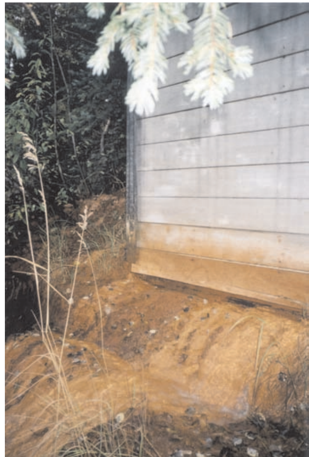
Photo 70. Red drainage flowing from the pump house at Island Mountain.
