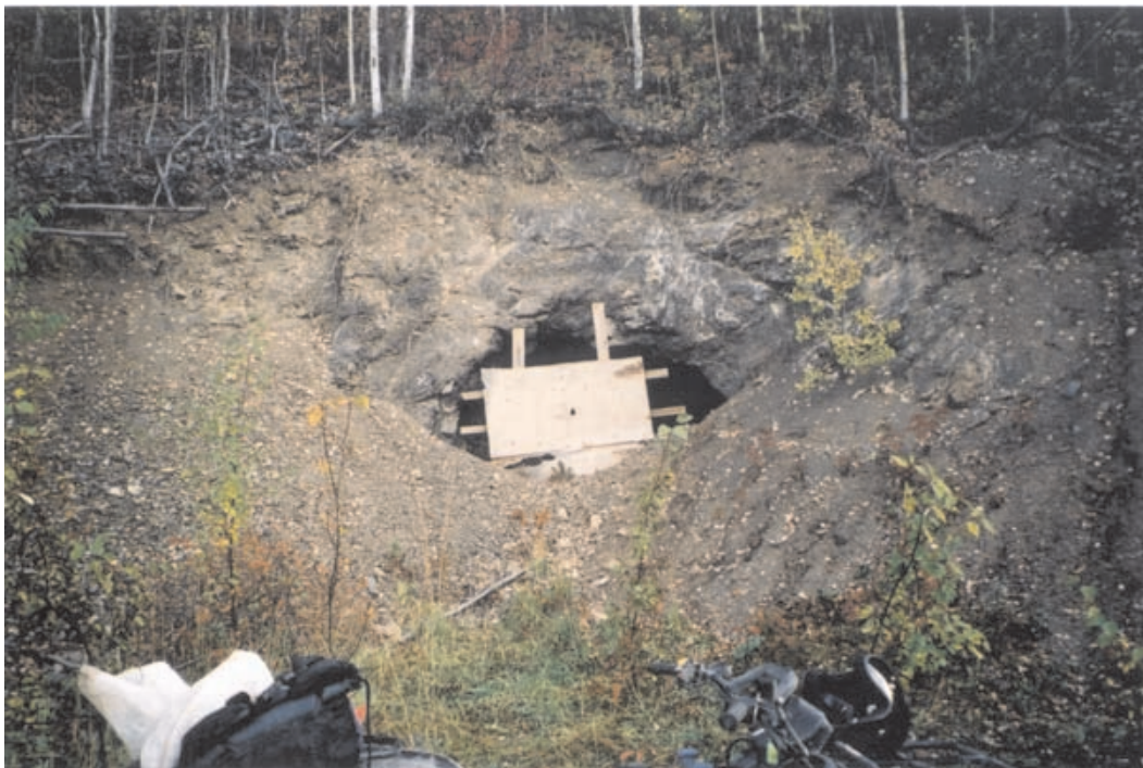
Photo 61. Northern portal at Snowbird mine containing a collapsed decline.
