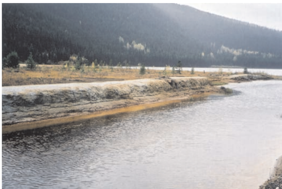
Photo 73. The Cariboo Gold Quartz tailings are submerged in Jack of Clubs Lake and the Willow River. Note the oxidized tailings along the bank of the Willow River.
