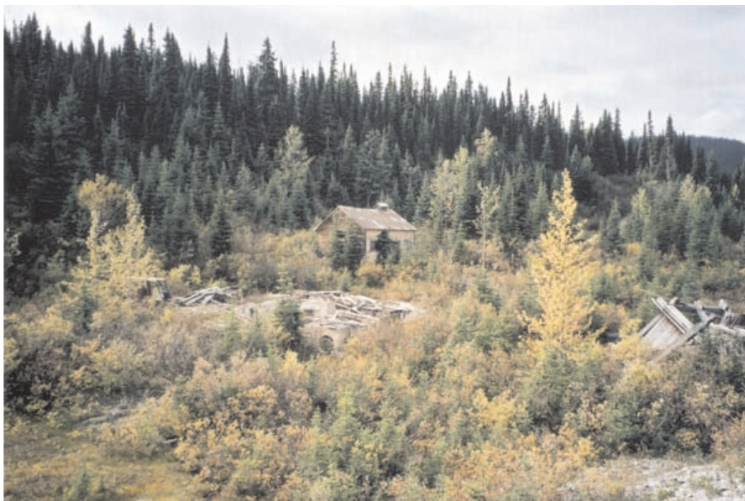
Photo 69. The shaft headframe and buildings (one is collapsed in the foreground) at Canusa mine site.
