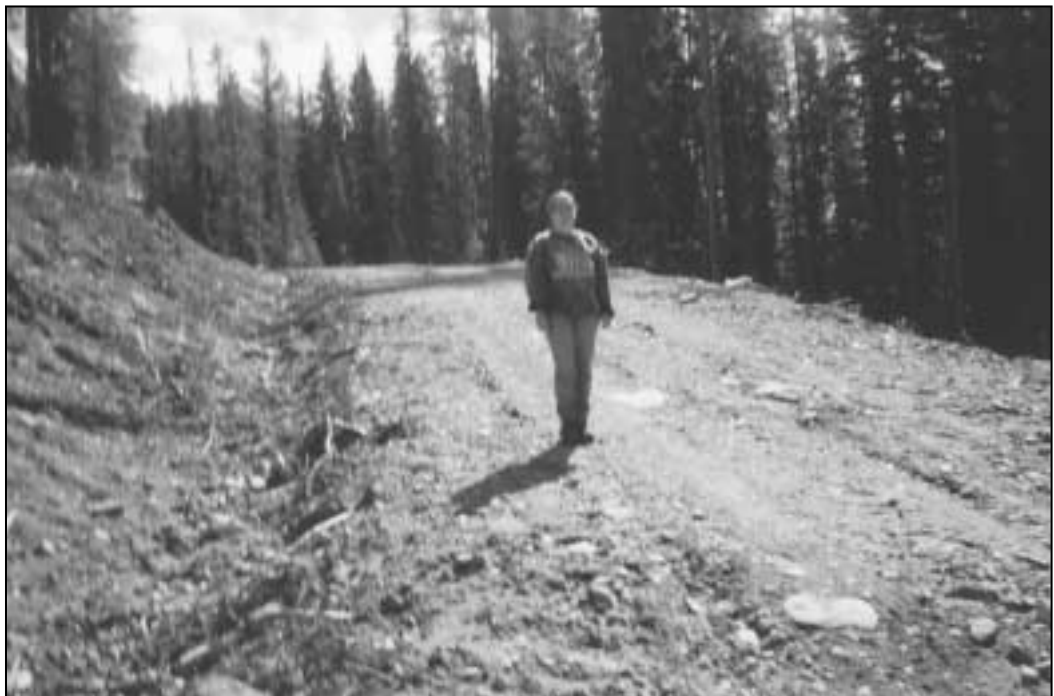
Figure A3.4. Example of sediment production class 4 (sediment production = 70 m 3 /km/yr).
