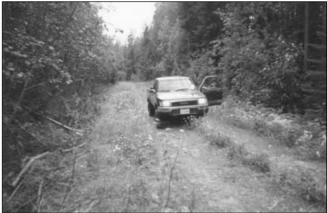
Figure A3.2. Example of sediment production class 2 (sediment production = 1.0 \text{ m}^3/\text{km}/\text{yr} ).
