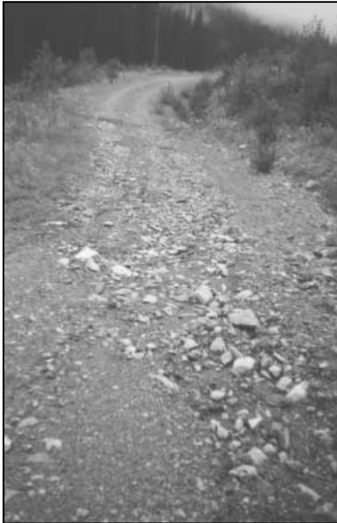
Figure A3.5. Example of sediment production class 5 (sediment production = 1,000 m 3 /km/yr).
