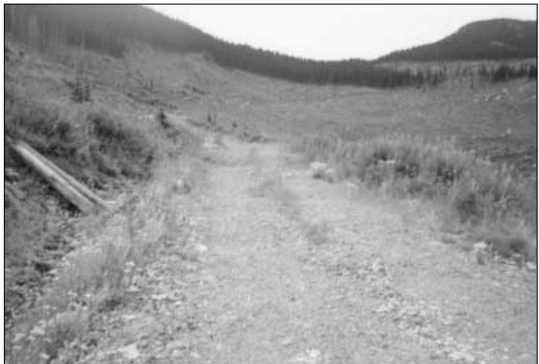
Figure A3.2. Example of sediment production class 2 (sediment production = 1.0 \text{ m}^3/\text{km}/\text{yr} ).
