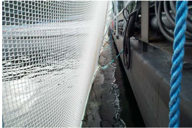
Net cage properly tied off at the water line.
