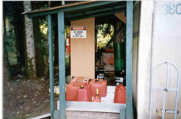
Gasoline containment and protection from precipitation
