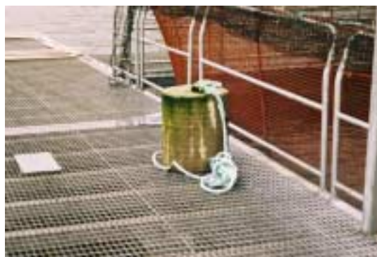
PHOTOGRAPH 3 - Typical concrete main anchor, used as external weight.
