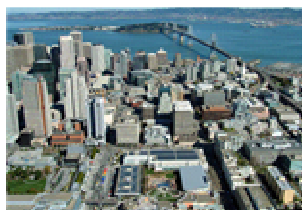
San Francisco's Moscone Convention Center solar power system uses Xantrex converters
