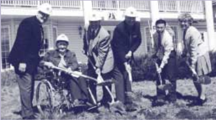
BREAKING GROUND IN KELOWNA — The Good Samaritan Society celebrates the start of construction of its 37 unit supportive seniors project in Kelowna. Pictured here (L-R) are: Dr. Archie Marzolf, Chair, BOD Good Samaritan Society; Rose Zukcht, Charter Volunteer Good Samaritan Society; Murray Ramsden, CEO, Interior Health Authority; Smiley Nelson, Kelowna City Councillor; Peter Chau, BC Housing; and Dyan Dunsmuir-Farley, Executive Director Care Services, Ministry of Health Services.
