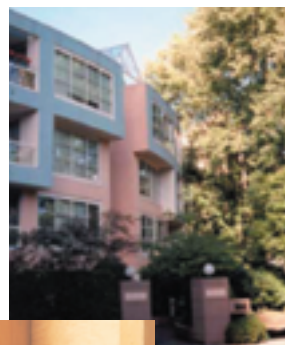
Photo courtesy of RDH Building Engineering Ltd.
