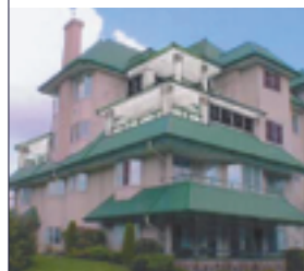
Photo courtesy of RDH Building Engineering Ltd.
