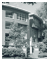
Photo courtesy of RDH Building Engineering Ltd.
