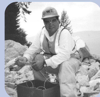
On site during Brilliant Expansion Project construction.
