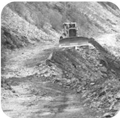
April 2003 - Bulldozer clearing access road at the Brilliant Expansion Project.
