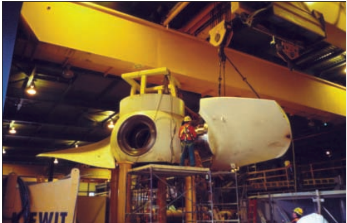
Installation of turbine runner at Arrow Lakes Generating Station
