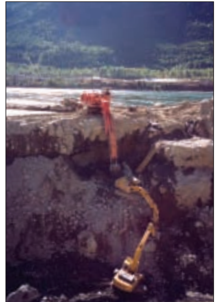
Excavating the approach channel
