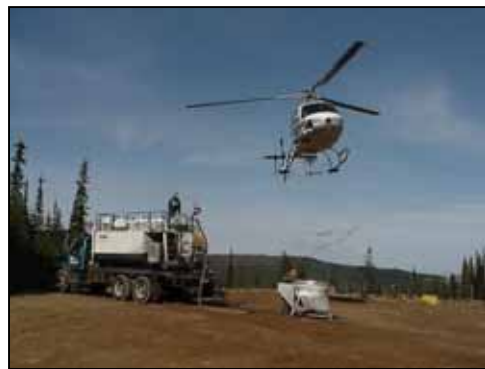
Hydroseeding with a helicopter. (picture from Mikolash, 2001)
