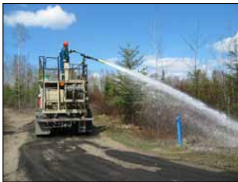
Hydroseeder being used to spray a foam line.
