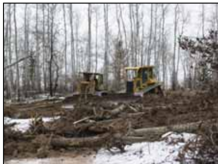
Two crawlers working together and a Nodwell with a hoe/excavator attachment.
