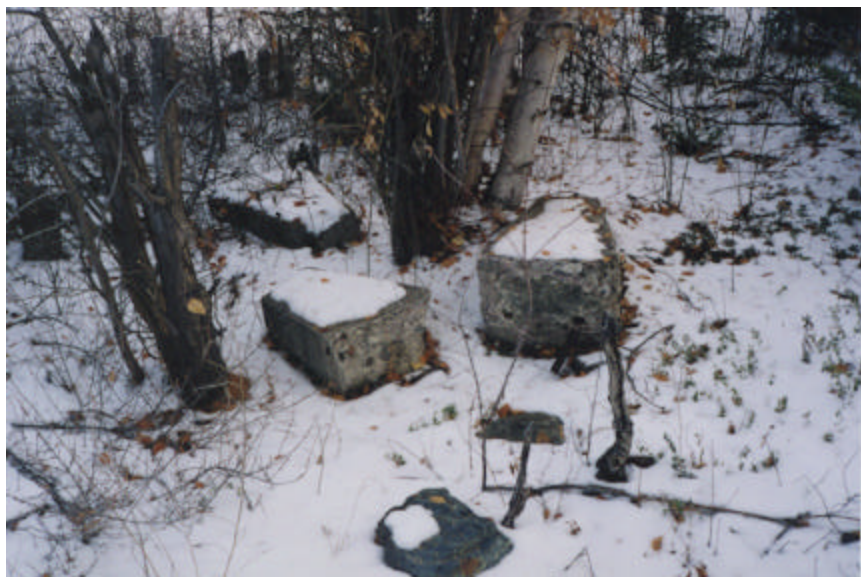
Photograph 6.18-3. Birch Lake Mine-Concrete Footings and Slab for Power Line-October 23, 2002.
