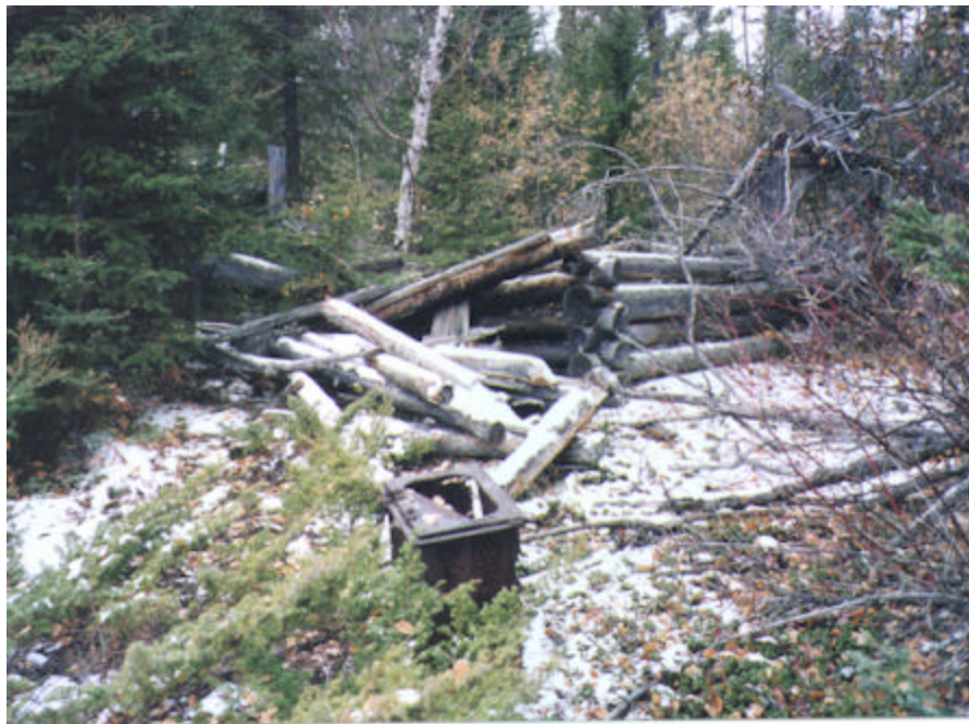
Photograph 6.12-3. Sonora Deposit-Collapsed Cabin-October 20, 2002.
