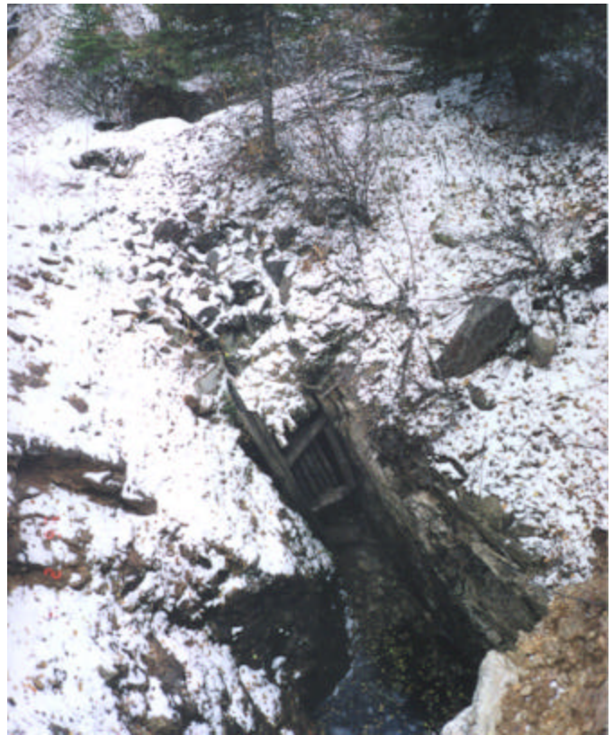
Photograph 6.7-7. Prince Albert Mine-Inclined Shaft and Stone-October 18, 2002
