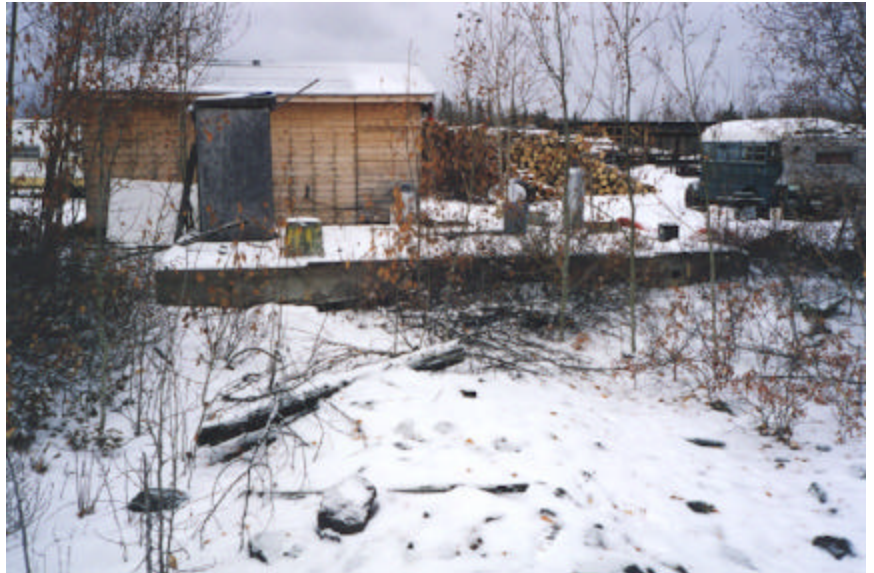
Photograph 6.29-8. Coronation Mine-Loading Platform-October 28, 2002.
