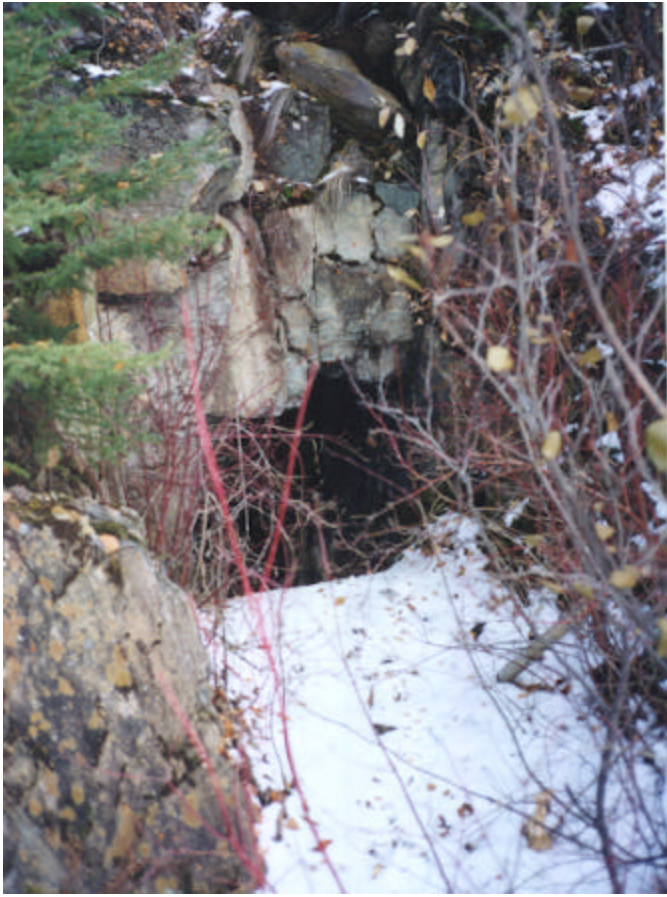
Photograph 6.15-4. Amisk Syndicate Mine-West Adit Portal-October 21, 2002.
