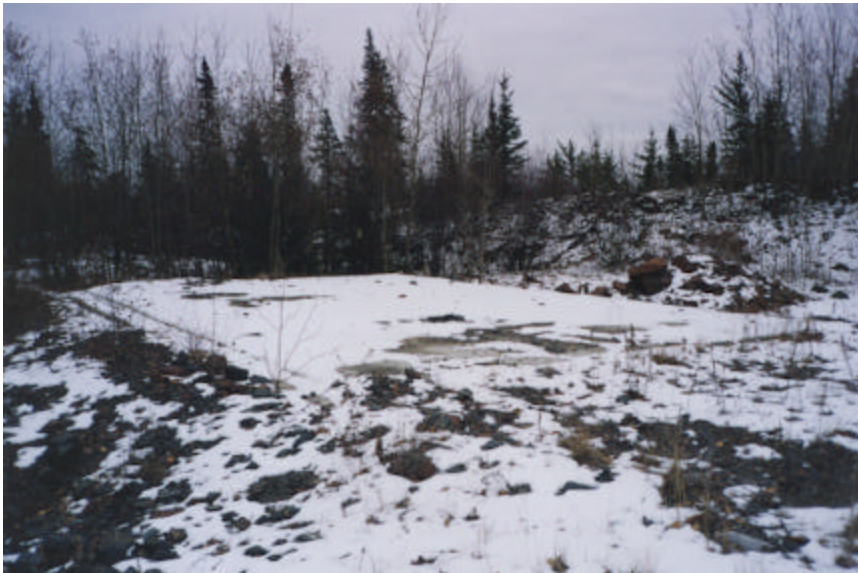
Photograph 6.23-6. Vista (Bootleg) Mine-Concrete Pad at Ventilation House-October 29, 2002
