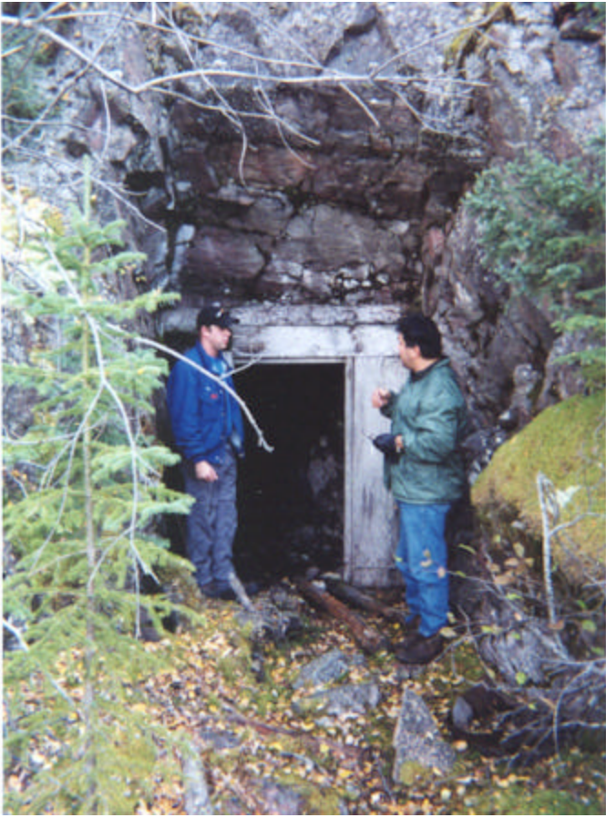
Photograph 6.2-1. New Mylamaque Site-Portal-September 30. 2002
