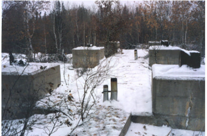
Photograph 6.29-5. Coronation Mine-Concrete Slab 'C'-October 28, 2002.
