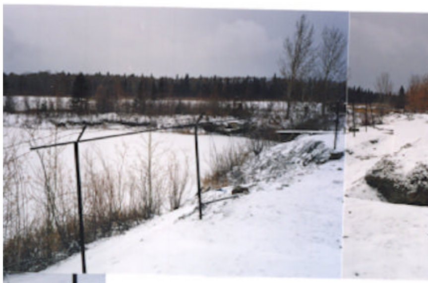
Photograph 6.29-3. Coronation Mine-Concrete Foundation 'A' (Mine Shop?)-October 28, 2002.
