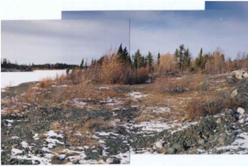
Photograph 6.19-3. Newcor Mine Site Concrete Ruins-October 24, 2002
