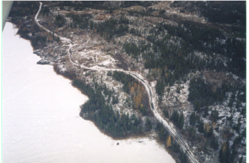
Photograph 6.19-2. Newcor Mine Site-Panoramic View-October 24, 2002
