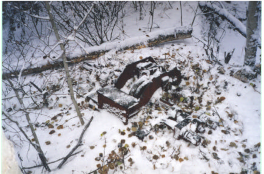
Photograph 6.24-8. Graham Mine-Collapsed Log Cabins-October 25, 2002.
