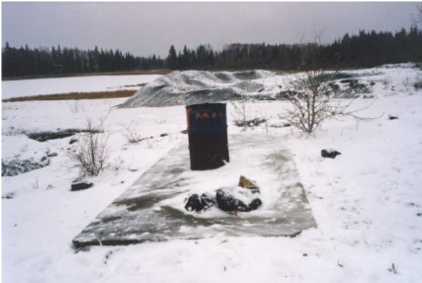
Photograph 6.29-6. Coronation Mine-Concrete Foundation 'D' (Shaft Area)-October 28, 2002.
