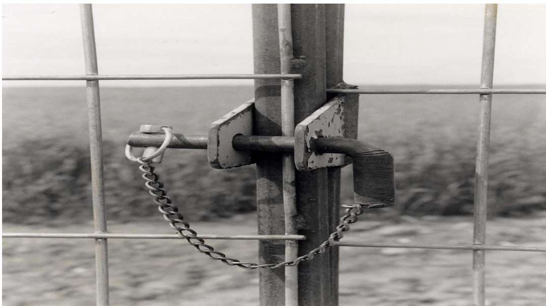
Figure 4. Simple Gate Latch Design
