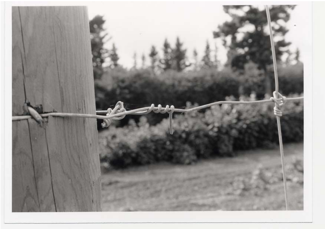
Figure 2. Example of an Efficient Method of Attaching Wire to Posts
