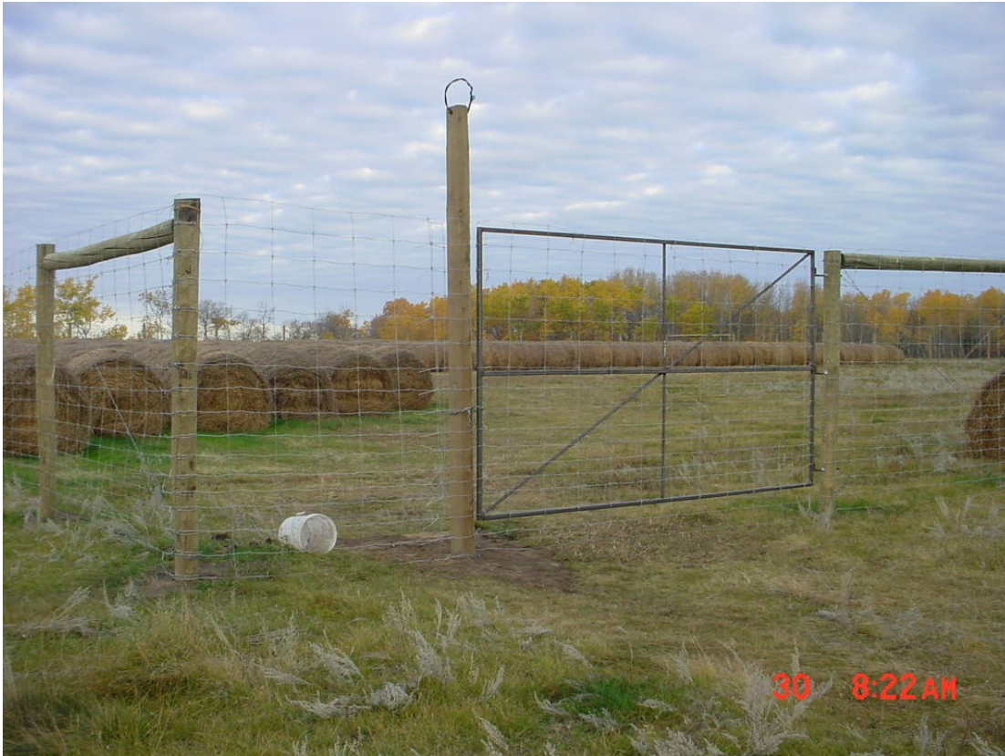
Figure 1. Examples of Corner Braces
