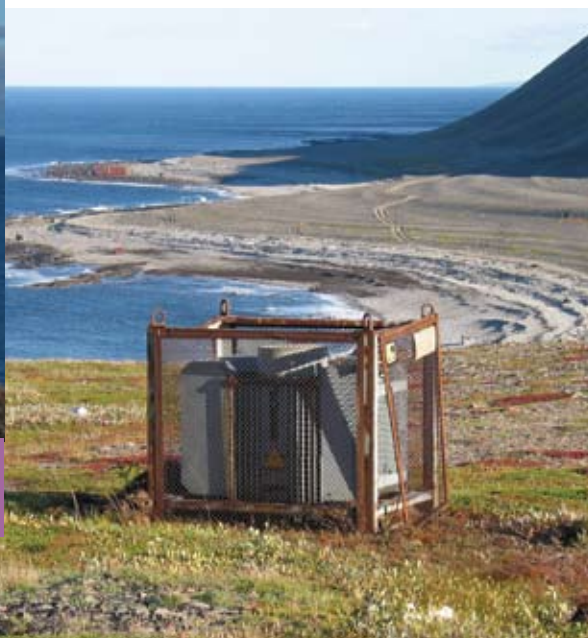
Highly radioactive materials that could be used in a "dirty bomb" are currently used to power lighthouses in the remote Russian north
