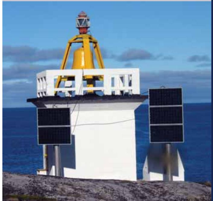
*Solar cell panels provide a sustainable alternative power source for lighthouses formerly powered by highly radioactive material. Photo Credit: County Governor of Finnmark (Norway)*
