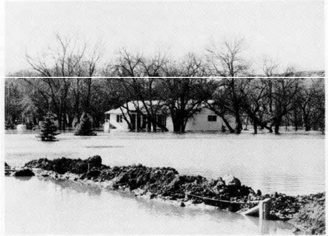
The consequences of building in a flood plain (photo credit: The SBDA).
