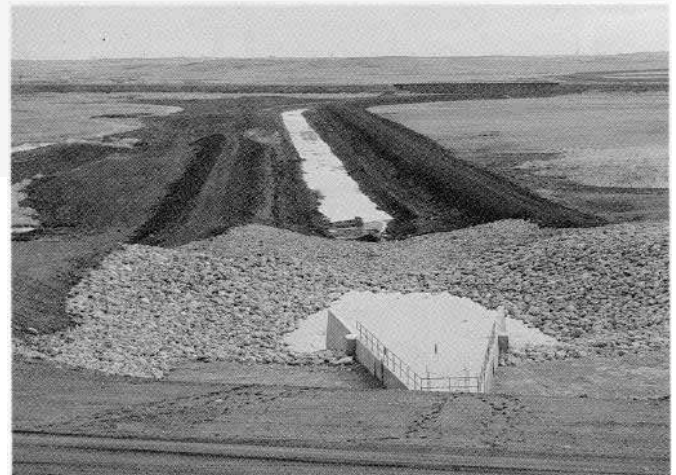
Rafferty Dam: low-level outlet and downstream channelization, April 1991 (photo credit: R. Riewe).
