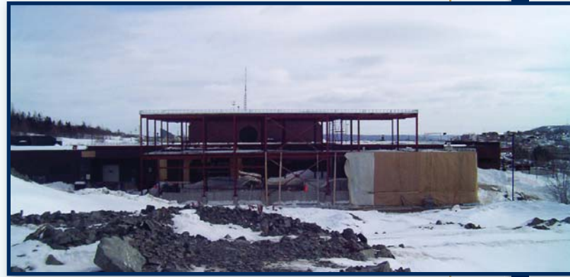
Construction of Clarenville long-term care facility
