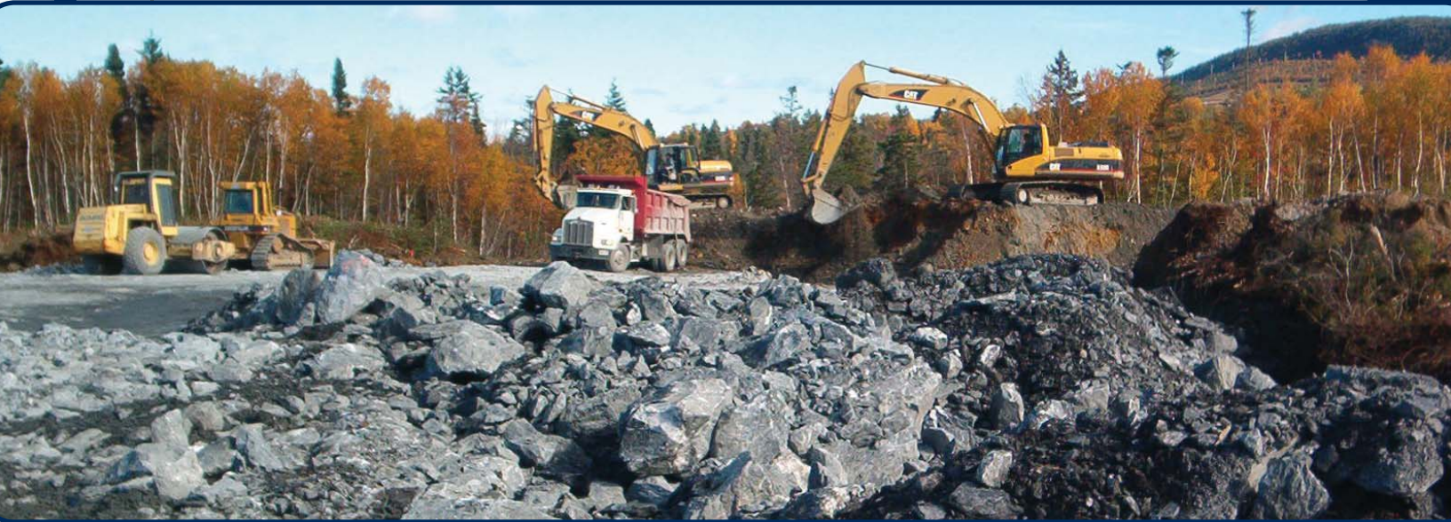
Site preparation for the Corner Brook long-term care facility
