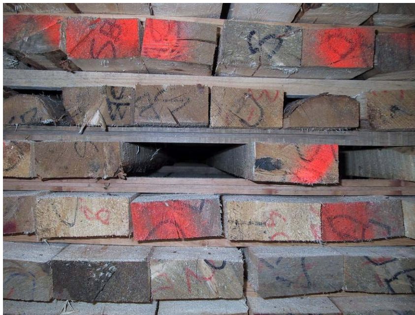
Figure 8: Picture showing clearance due to sawing variation and resulting twisted boards.
