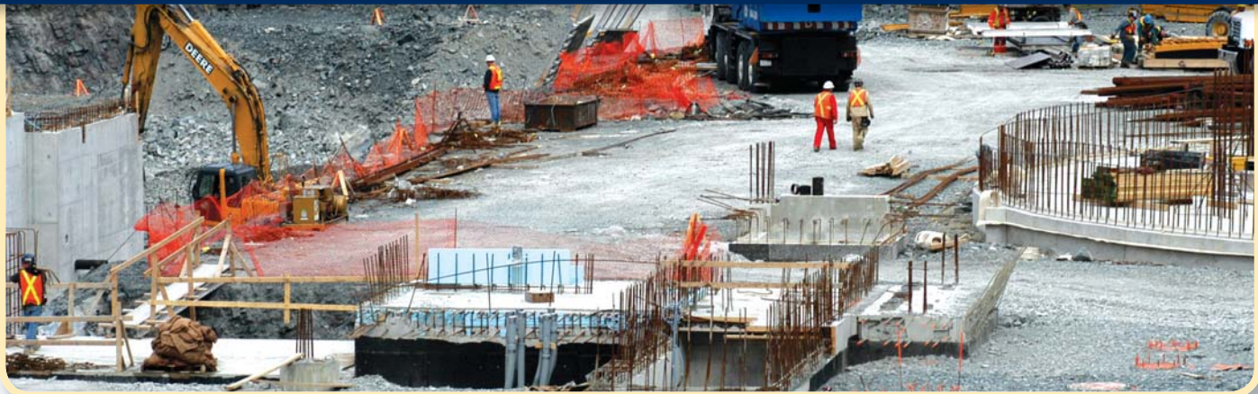
Construction of Riverhead Waste Water Treatment Facility—St. John's
