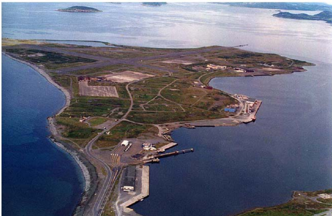
Figure 4 Argentia Hydromet Demonstration Facility Site
