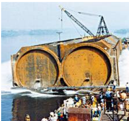
Figure 6.7: Launching Steel Element, Fort McHenry Tunnel, Baltimore, MD
