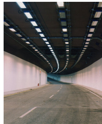
Figure 6.5: Completed ITT, River Lee Tunnel, Ireland
