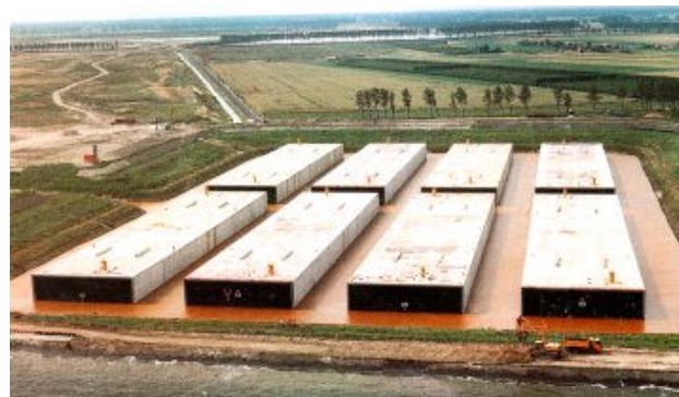
Figure 6.1: ITT Elements in Casting Basin, Liefkenshoek Tunnel, Belgium
