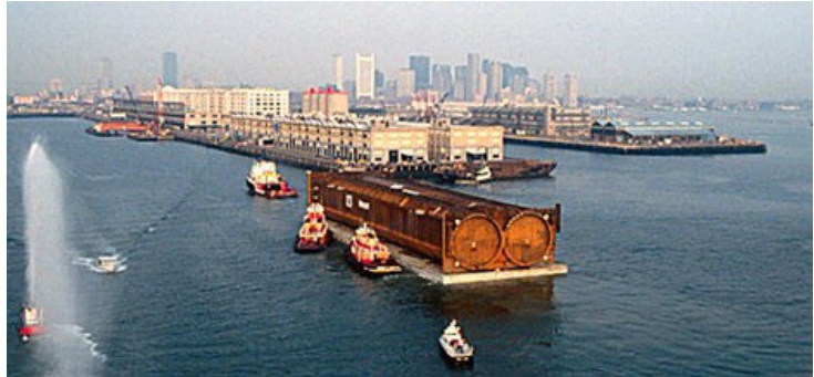
Figure 6.8: Transport of Steel Element, Ted Williams Tunnel, Boston, MA
