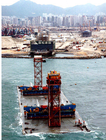
Figure 6.3: Element prior to Immersion, Western Harbor Crossing, Hong Kong
