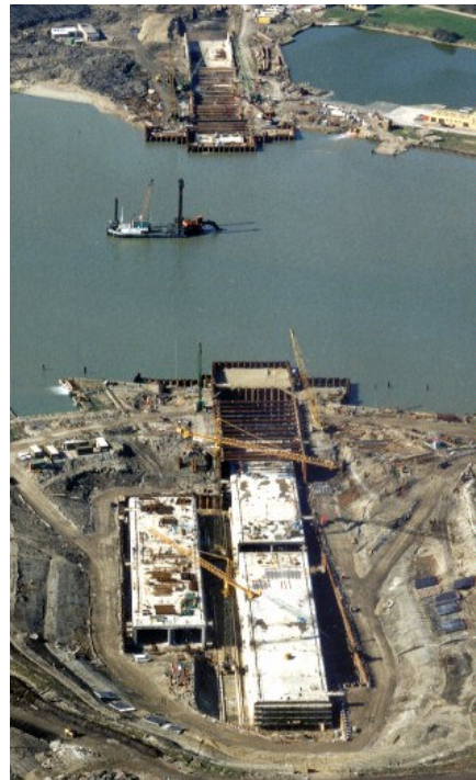
Figure 6.2: Tunnel Construction & Channel Dredging, Medway Tunnel, UK
