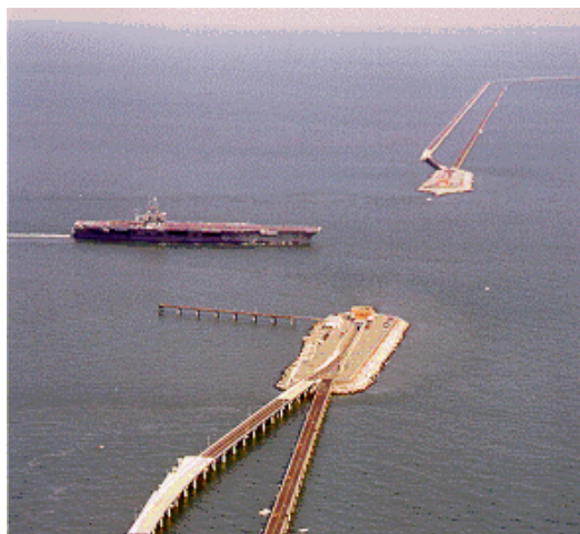
Figure 2.5 - Chesapeake Bay Bridge Tunnel
