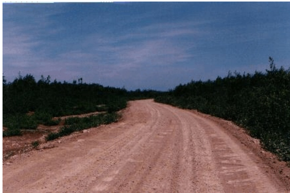
Forest Resource Road Construction
