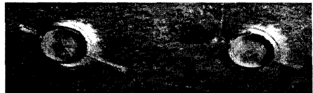
Figure 4: (a) Edge of Light image of two rivets from a Boeing 737. There are two cracks extending from each rivet. The rivet heads are about 7 mm in diameter.
