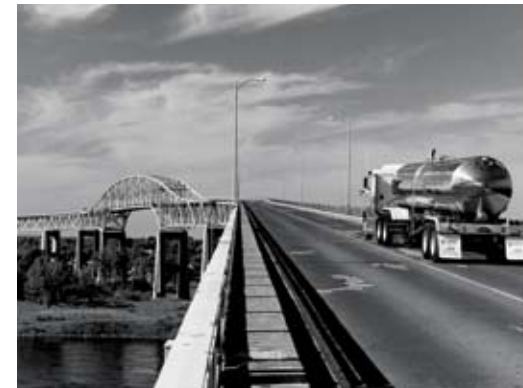
↑ The Seaway International Bridge
