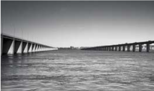
↑ The Champlain Bridge Ice Control Structure
