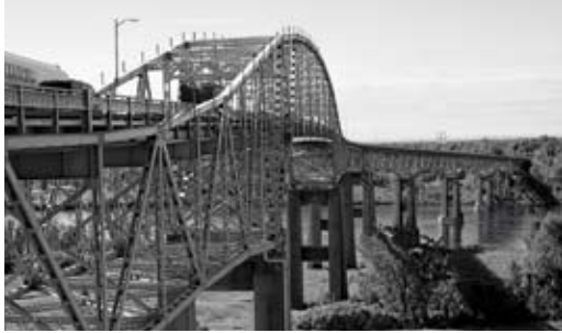
↑ The Seaway International Bridge
