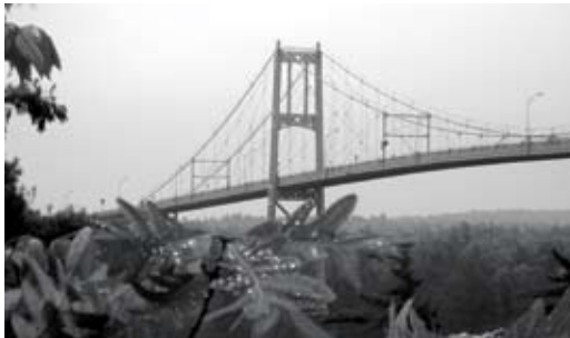
↑ The Thousand Islands International Bridge
