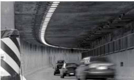
↑ The Melocheville Tunnel
