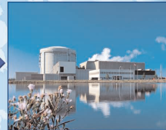
Pt Lepreau 680 MWe In-service: 1983 Pointe Lepreau 680 MW(e) En service : 1983
