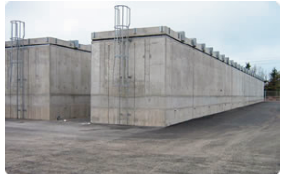
Construction of the SRWMF vaults and canisters, which will house radioactive waste removed from the retube operations during the generating station's refurbishment, was completed a year ahead of schedule.
