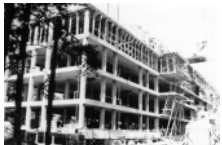
Construction of Forest Hall, 1958
