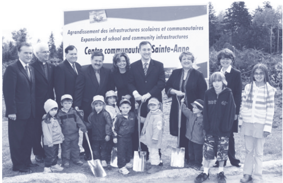
Josée Verner and New Brunswick Premier and Minister of Intergovernmental Affairs, Bernard Lord, at the start of construction to expand the Centre communautaire Sainte-Anne.
