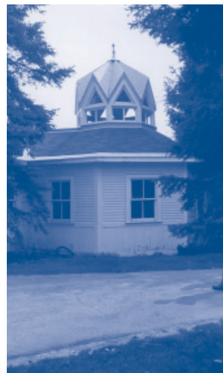
Former Rideau Hall dairy (around 1979)
