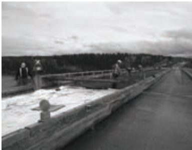
Workers replace the Teslin River bridge deck.
