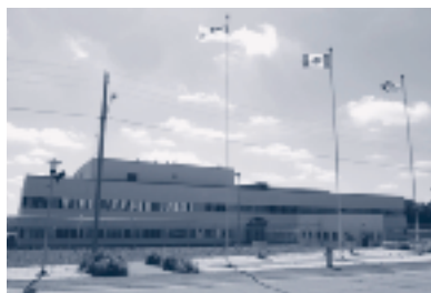
New above-ground complex at Canadian Air Defence Sector, North Bay, Ontario
