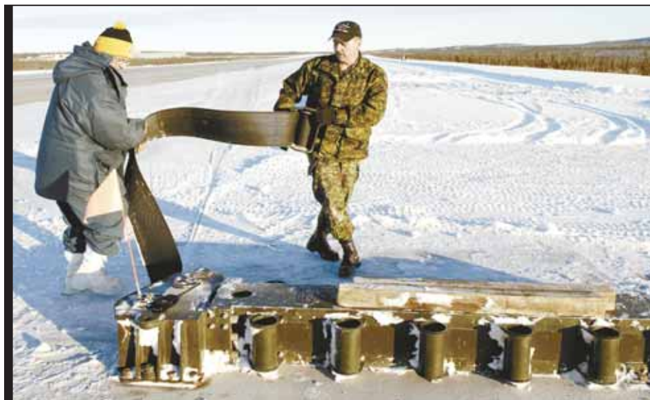
John McDonald and Sgt Bernie MacInnis reset the arresting cable at the Inuvik Airport after a CF-18 aircraft engaged the cable on landing. Sgt MacInnis is a refrigeration and mechanical systems technician from 4 Wing Construction Engineering, 4 Wing Cold Lake.
