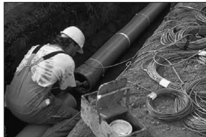
Measuring the magnitude of forces acting on water mains
