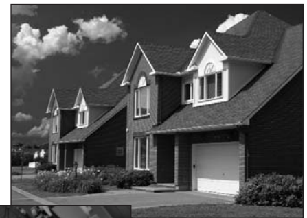
Twin research houses at the Canadian Centre for Housing Technology
