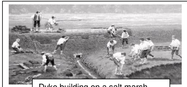
Dyke building on a salt marsh
