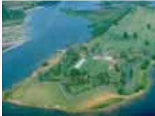
Fort Lennox, Quebec Early 19th Century Fortifications
