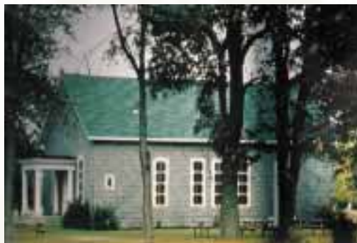
Buxton Settlement, Ontario Schoolhouse in Farming Community Established by Underground Railroad Refugees
