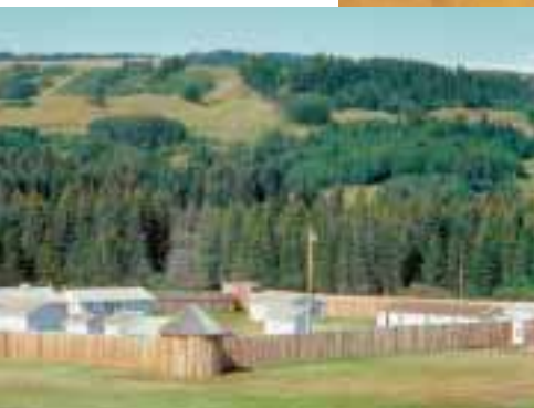
Fort Walsh, Saskatchewan Early North-West Mounted Police Post
