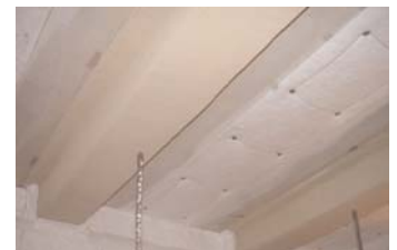
Beam slab assemblies before testing
