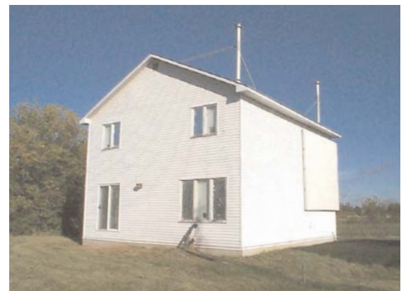
NRC Two-Storey Research House – back
