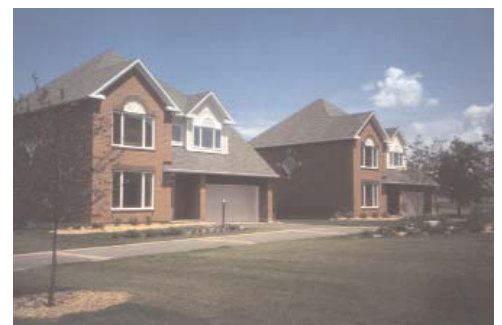
Twin Research Houses at the Canadian Centre for Housing Technology
