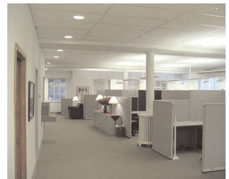
Office with individually controlled lighting (dimming control)
