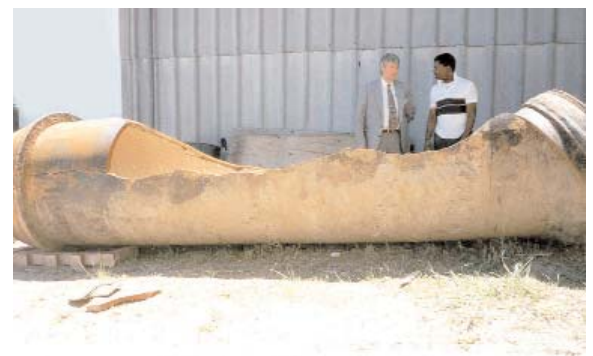
Failed cast iron transmission main
