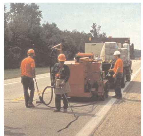
Workers apply crack sealant to pavement
